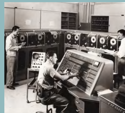
From past to present, Livermore has employed the most powerful computer systems available to support stockpile stewardship design and test efforts. Left: The Univac, Livermore’s first supercomputer, had 5,600 vacuum tubes, a 6-kilobyte memory, and a code stored on magnetic tape. Right: LLNL’s newest supercomputer system, Sierra.
